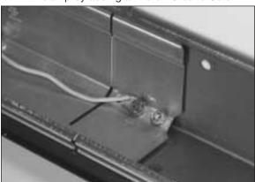
Step 4. Where the Adjust-to-Fit Coupling<sup>™</sup> is too long, the Coupling can be trimmed at the notch and broken into a smaller piece. Remove Screw from larger section and place in the open hole on the smaller piece.
