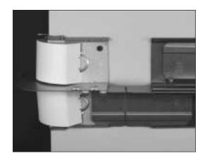
**Step 2.** Coupling can slide in from the end of the Raceway or snapped in as shown.
