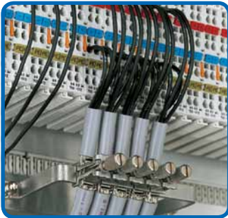
Installation on U-shaped copper busbar
