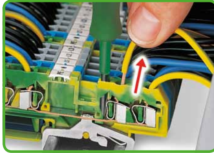
Removing conductor via screwdriver.
