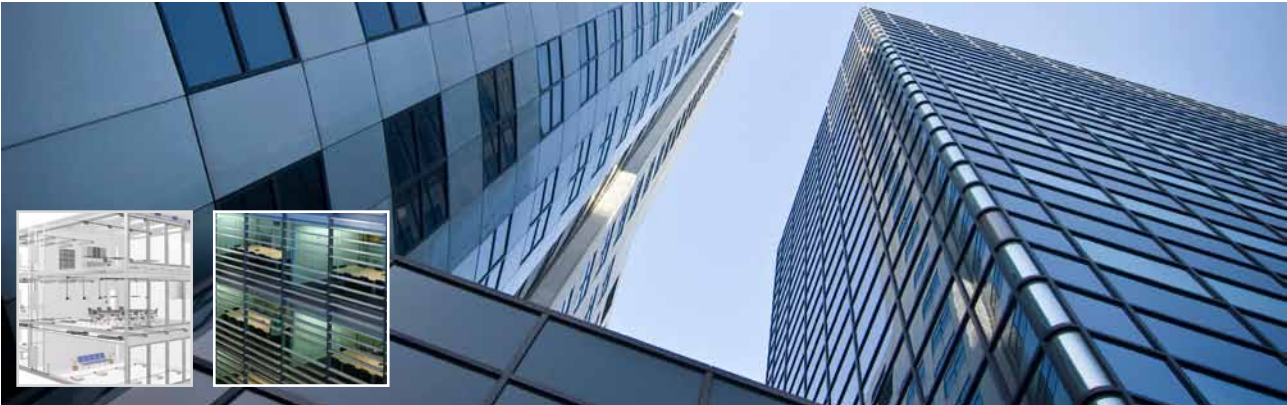
Building installation and automation
