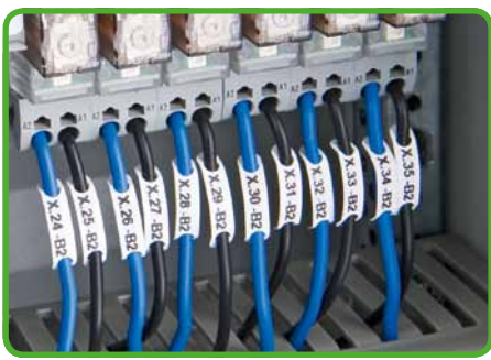
Conductor Marking for Thread-On Mounting
