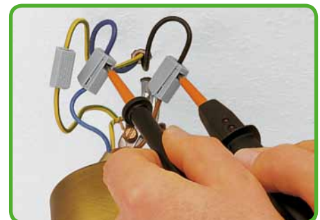
Testing through separate test slot.
