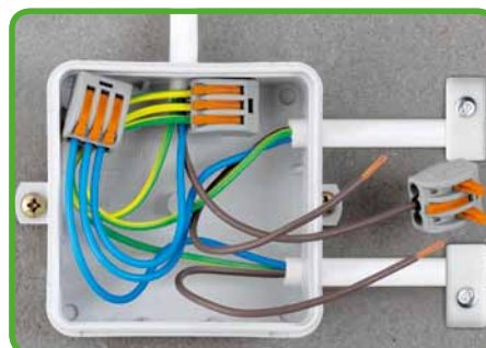
Wiring fine-stranded conductors in a junction box.
