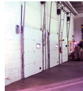
Sturdy and safe wall fixtures light these loading docks
