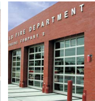
Fixture with red globe makes a great signaling device at firehouses...
